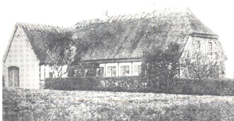
Kold's folk high school in Ryslinge. The buildings have been preserved.
