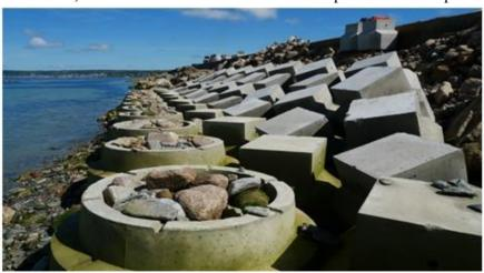
The aim of this new ACCROBERM<sup>TM</sup> II block is to provide two functionalities, i.e., both a toe block and a support for biodiversity by providing new habitats including microhabitats.
