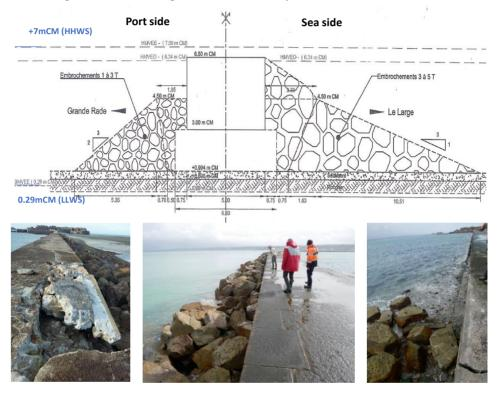
The Eastern breakwater was damaged on several occasions and the most recurrent problem is missing rocks, observed especially on the seaward side, where the rock slope protection has been either partially eroded or completely removed. It is not uncommon to see large rocks (3-5t) that have been extracted and transported far away from the armour layer.
