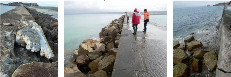
The Eastern breakwater was damaged on several occasions and the most recurrent problem is missing rocks, observed especially on the seaward side, where the rock slope protection has been either partially eroded or completely removed. It is not uncommon to see large rocks (3-5t) that have been extracted and transported far away from the armour layer.
