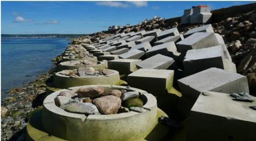
The aim of this new ACCROBERM™ II block is to provide two functionalities, i.e., both a toe block and a support for biodiversity by providing new habitats including micro-habitats.
