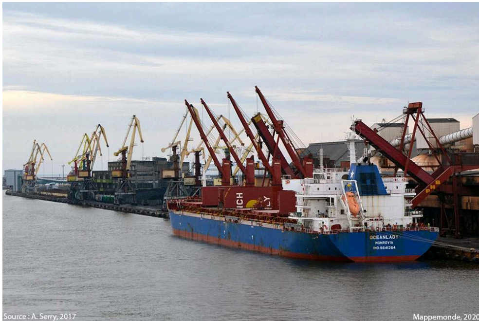
Figure 10. Le terminal charbonnier de Ventspils
