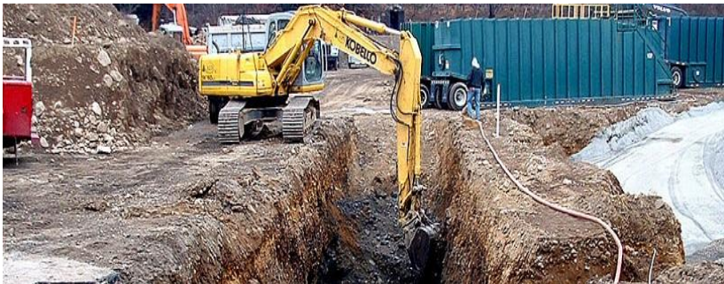
Soil excavation for ex-situ treatment
