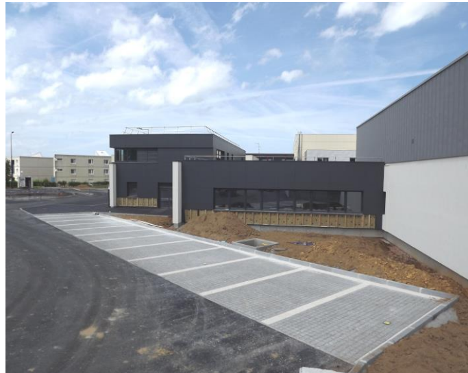
Fig 2. Parking spaces made with pervious concrete pavers – ESITC Caen, Epron, France
